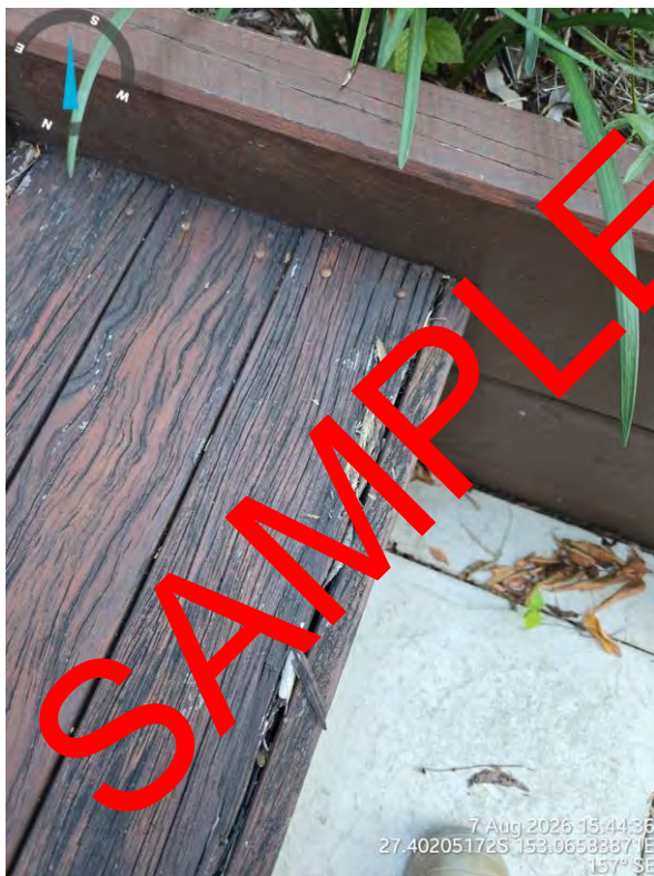
P12 - Close-up showing breakdown and loss of timber fibres at the edge of a horizontal member.
