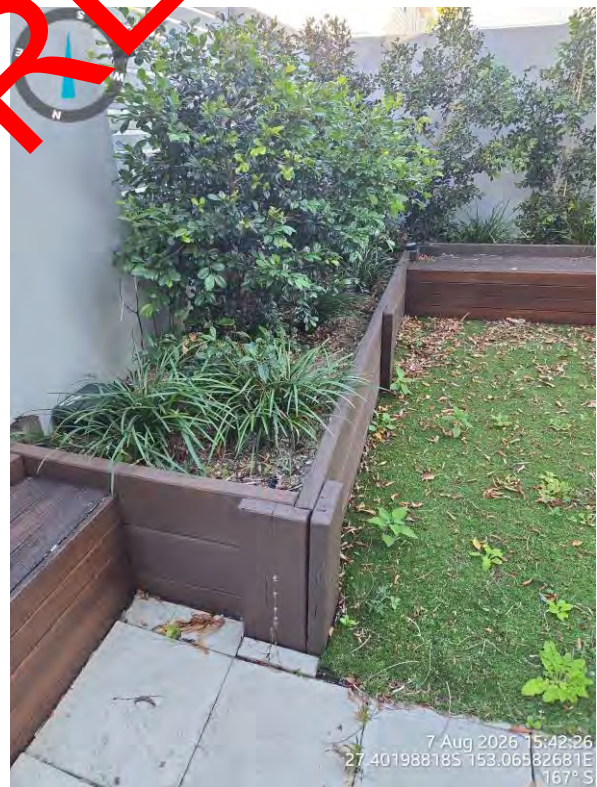
P05 - Cracked and deteriorated exposed top of timber post/block.
