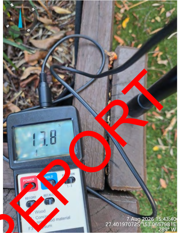
P04 - Moisture reading of 13.8% at an external timber junction.
